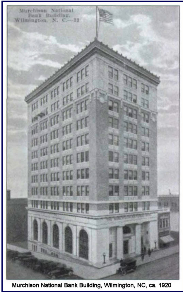
Fig. 3. Murchison National Bank building, Wilmington, NC, circa 1920.
